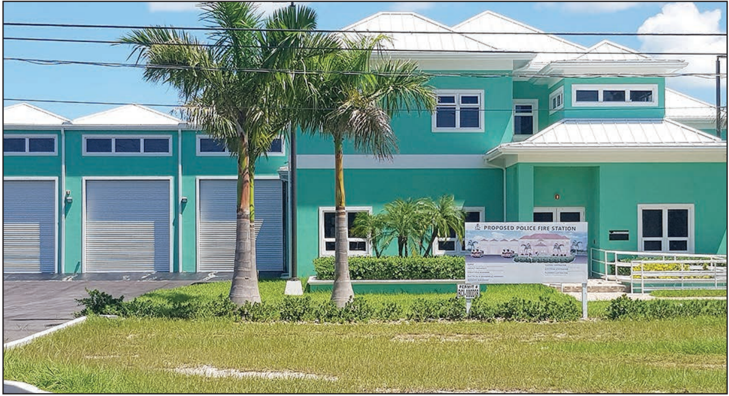
UNOPENED — The Fire Services Station, located on Cathedral Boulevard (formerly Settler's Way) remains closed despite the completion of the construction of the facility more than a year ago. (PHOTO: JAIMIE SMITH)
